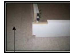
Large notch-out on side boxout faces up.
