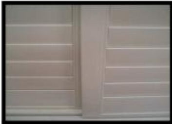
Check center stiles for alignment.
