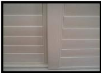
Check center stiles for alignment.
