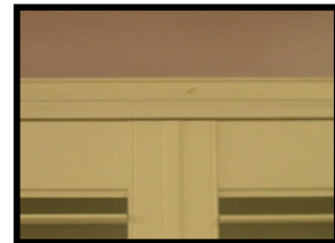
After racking of shutter, panels should line up.
