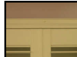
Double Check panels before securing.
