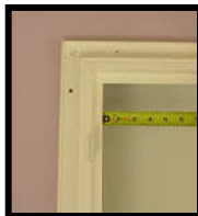
A tape measure can help space your shutter evenly around window.
