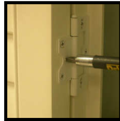
Loosen screws on panel hinge. Do not remove completely.
