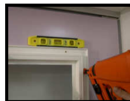
Only secure one nail into the top right frame.
