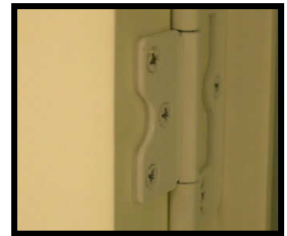
Hinge spacer installed
